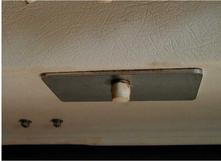
Figure 7 Old eyebolt backing plate, aft starboard.
